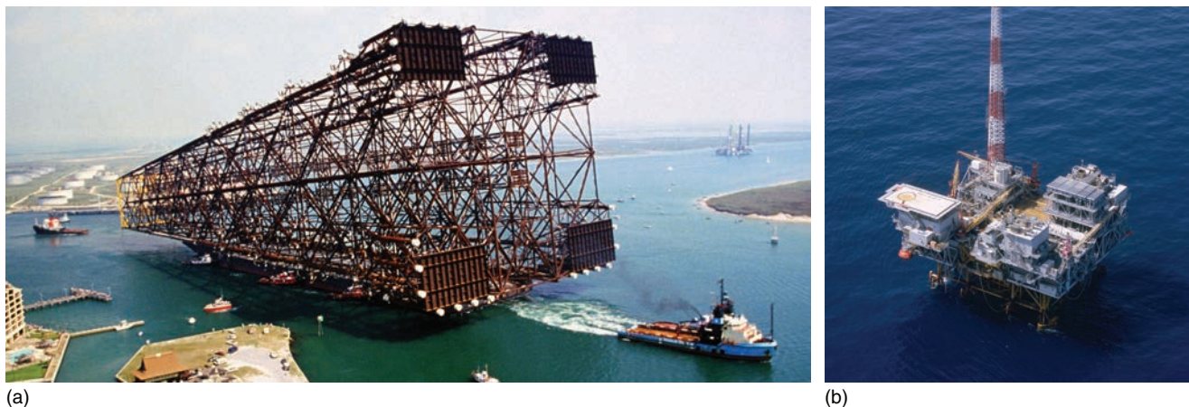
Figure 9. The Bullwinkle jacket was towed (a) to its location and installed so the topsides (b) could be set on the jacket in 1353 feet of water in the Gulf of Mexico. (Reproduced with permission. © Shell, 2016.)
