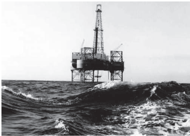
Figure 5. The first jackup rig, Scorpion , was built for Zapata Offshore Company for use in the Gulf of Mexico. (Reproduced with permission. © Rowan Companies.)
