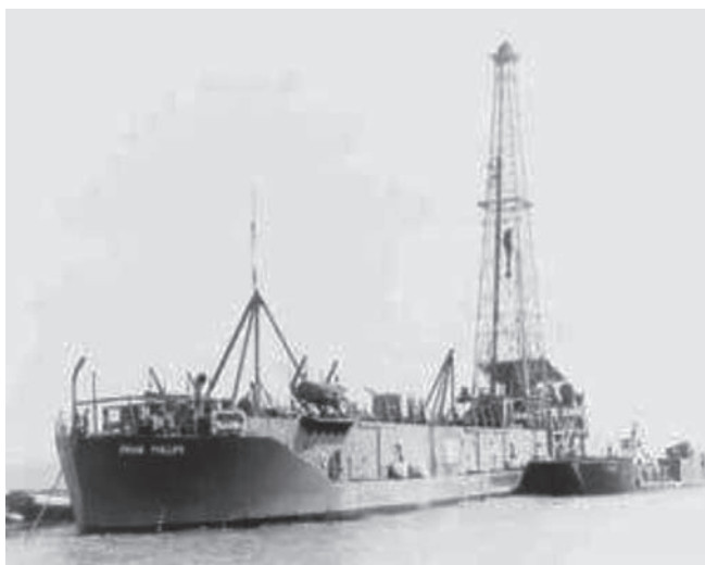
Figure 4. Kerr-McGee drilled in 18 feet of water using a drilling tender, Frank Phillips , a converted US Navy barge. (Photo Courtesy of Kerr-McGee.)
