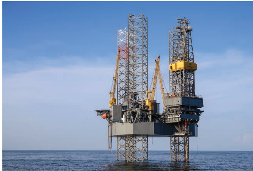
Figure 6. The Joe Douglas , an independent leg cantilever jackup built in 2011, can drill in 350 feet of water. (Reproduced with permission. © Rowan Companies.)
